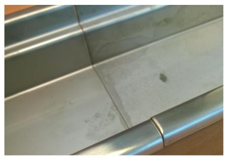
5. Once installed, seal join with approved aluminium coloured sealant.
